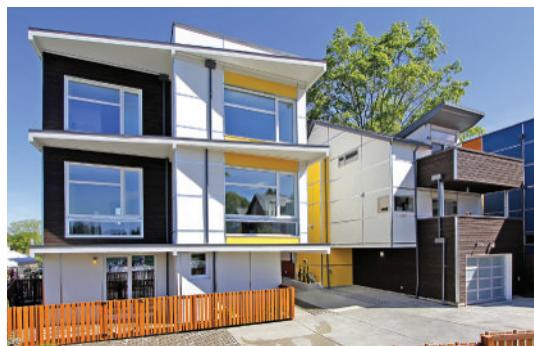
The flat roofs provide an ideal location for roof-top decks and solar panels, supported by 18-inch roof trusses that provide space for a combination of 2 inches of closed-cell spray foam and more than 16 inches of blown cellulose delivering an R-60 insulation value. Double-stud 14-inch-thick walls allow for R-45 of blown cellulose.
